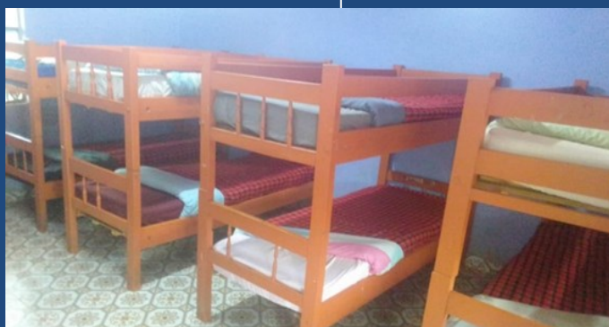
Section of renovated Dormitory at Rehema Girls' Home
